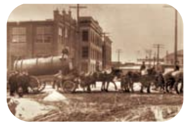
The 'early days' at Union Pump Company, moving a boiler
